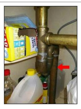
when water is done draining, air may be sucked in from the sink basin to fill the top loop, causing a gurgling sound
